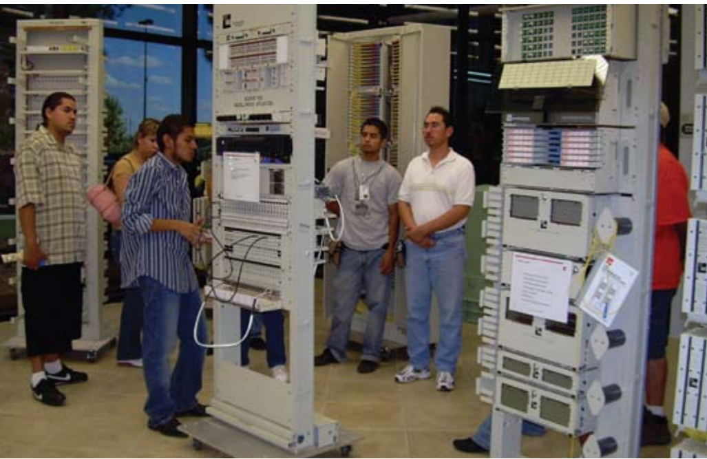
ADC employees are given a tour by Rafael Saledo, Systems Engineer Associate, of our new product demonstration room in Santa Teresa, New Mexico. This is one of many global product demonstration rooms that educate customers and employees on our product portfolio.
